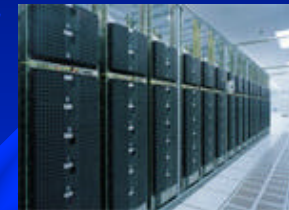
Data Center (Server Farm)
